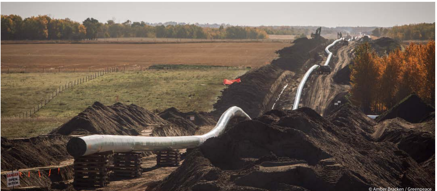
Enbridge's Line 3 Expansion in Canada, September 15, 2016.
